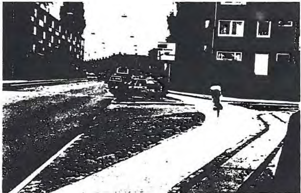
Figure 4.6 Staggered cycle track.
