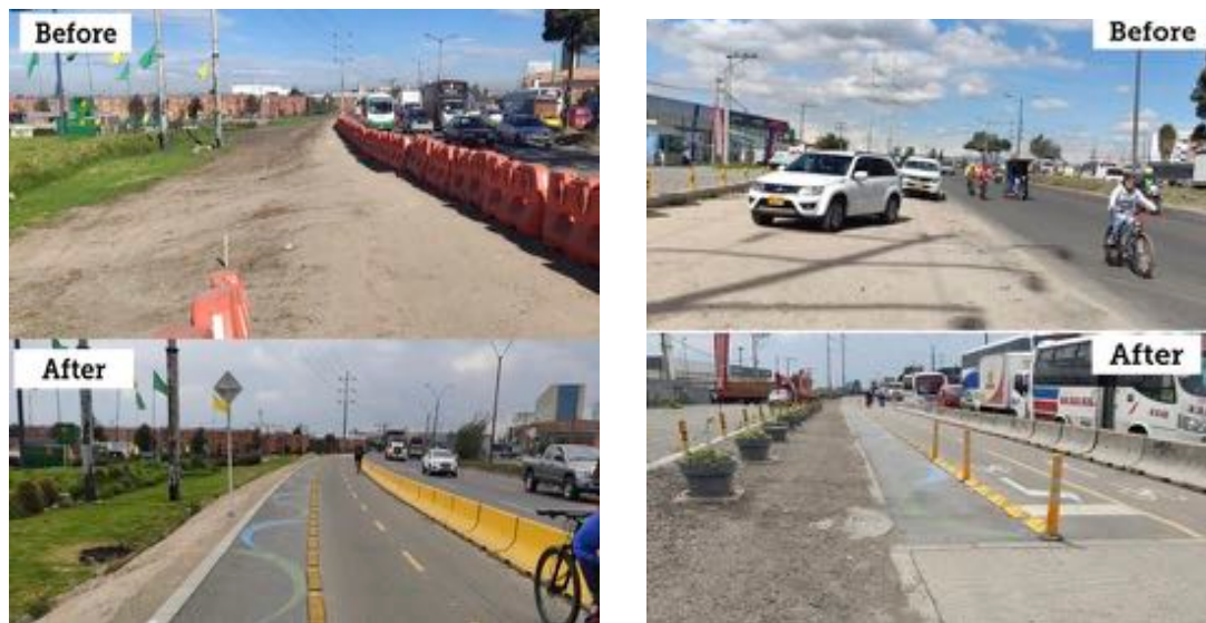
Figure 1.3.5. Cycling infrastructure in Bogota
