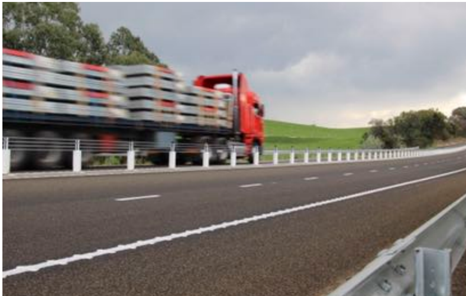
Figure 2.2.2. Barriers installed under the Safe System Road Infrastructure Top 20 Program
