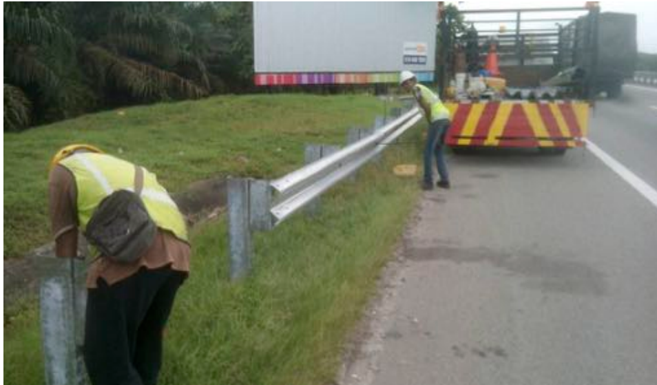
Figure 2.4.4. Safety improvements by PLUS Malaysia Berhad
