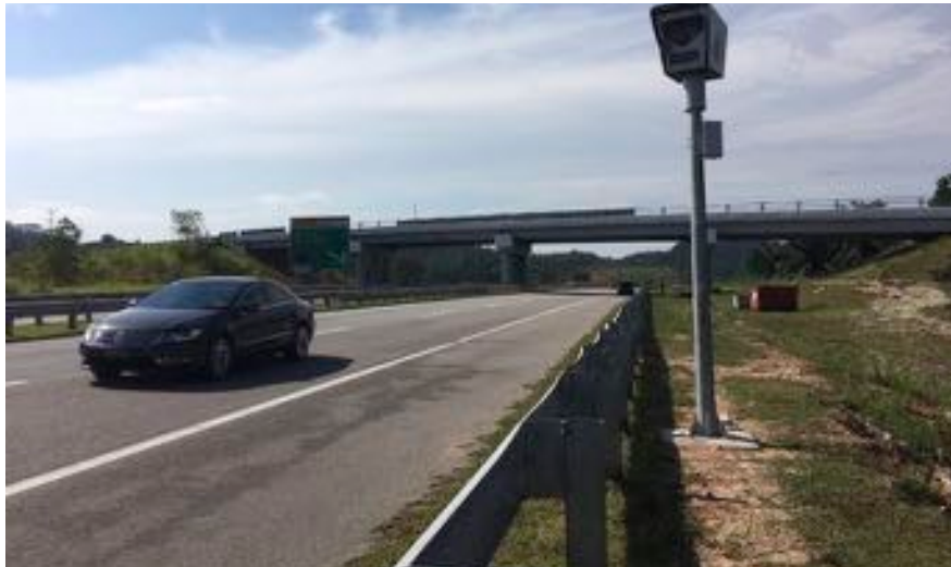
Figure 2.4.2. Automated Enforcement System Camera for Speeding
