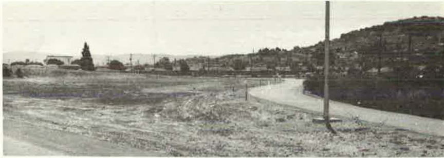
Figure 19. Except for the light standard, there is ample unobstructed recovery space here.
