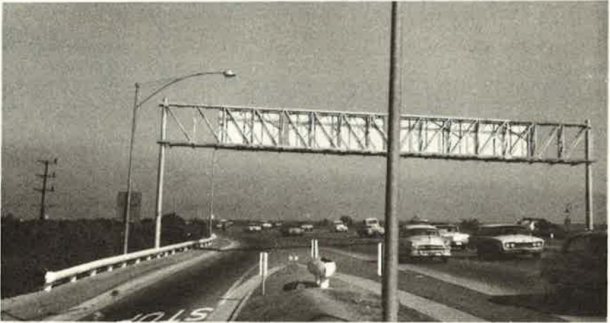
Figure 16. Why the guardrail in the gore?
