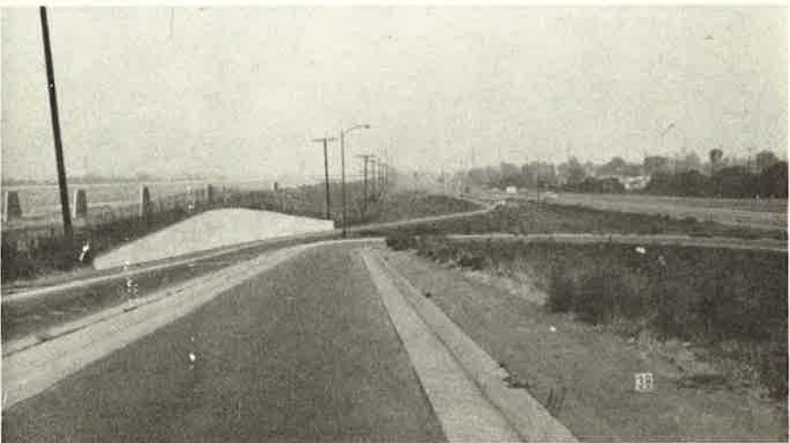
Figure 17. Curbs used for drainage, delineation and barrier.
