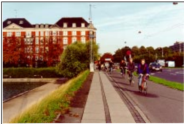
Cycle track with verge between cycle track and roadway Photo: The Danish Road Directorate
