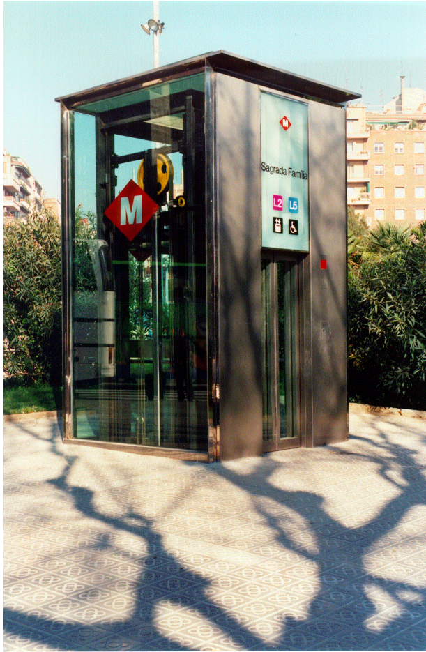
Access to the vestibule of a metro stop - Line III - in Barcelona (Spain)
