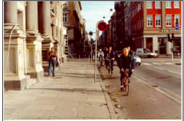
Cycle track (track and roadway separated by a kerbstone) Photo: The Danish Road Directorate
