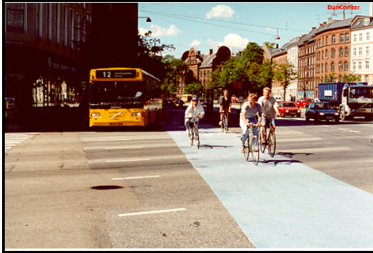
The blue cycle lane continues through the junction as a cycle crossing Photo: The Danish Road Directorate
