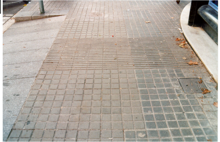
Pavement adapted for blind people indicating the location of a zebra crossing
