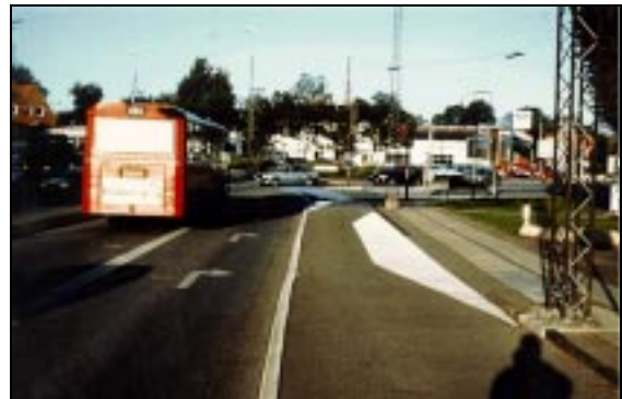
Interrupted cycle track at junction Photo: The Danish Road Directorate
