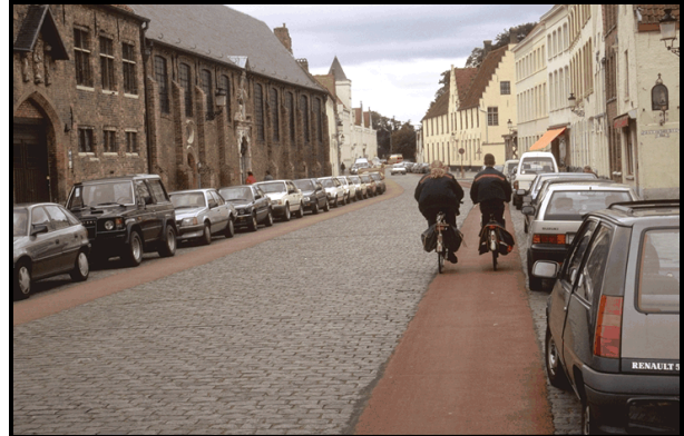
Non-compulsory cycle lane in cobbled street
