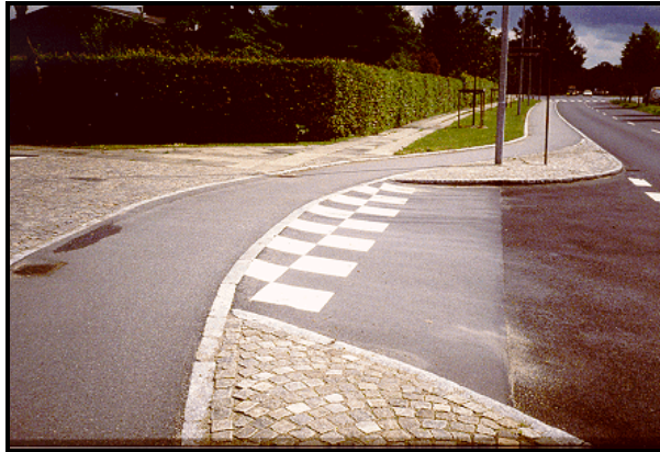
T-junction after reconstruction Photo: The Danish Road Directorate
