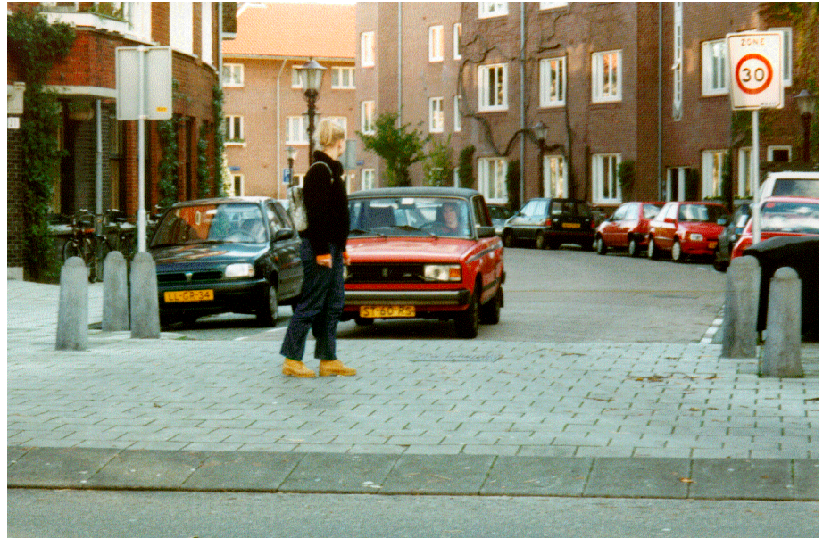
Exit construction in Amsterdam-Zuid
