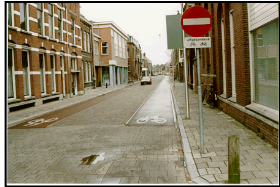
Partial one-way traffic with spacious profile Photo: SWOV, Institute for Road Safety Research, A. Vis
