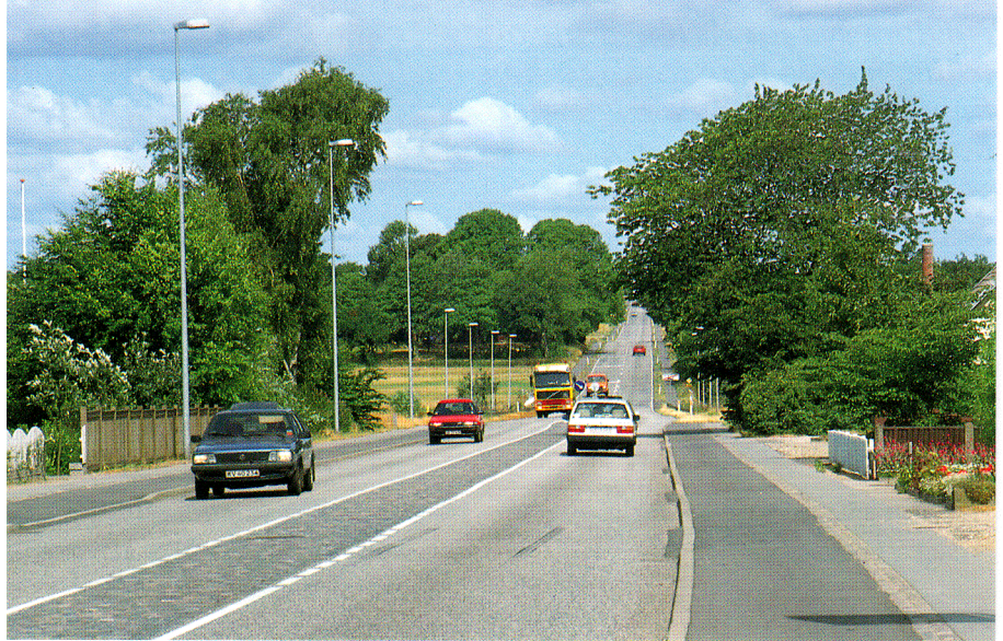
The reduced width of the carriageway lowers speeds and the granite-set band functions as a waiting zone for left-turning cars. /7, p. 127/.
