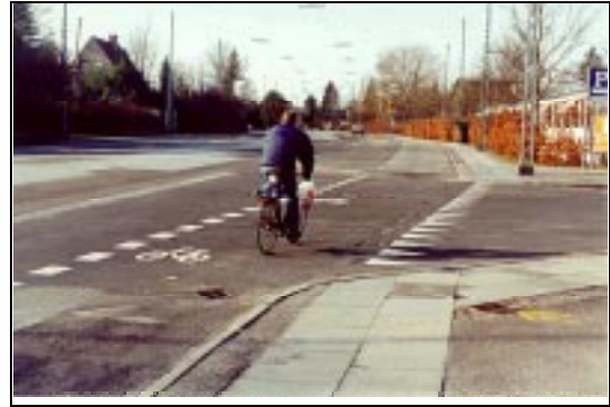
Crossing – Left hand edge Photo: The Danish Road Directorate
