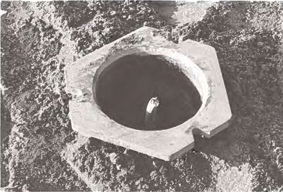
Figure 1. The slip design was developed so that the column could separate from the root section in an impact under controlled conditions. For this, the root section and the column were fitted with flanges which can be bolted together. The root-section flange should be about 3 cm above ground level.
