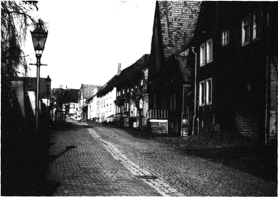
Figure 16: Village street (Borgentreich /Borgholz) reconstructed in an exemplary manner, formerly used locally as bypass route
