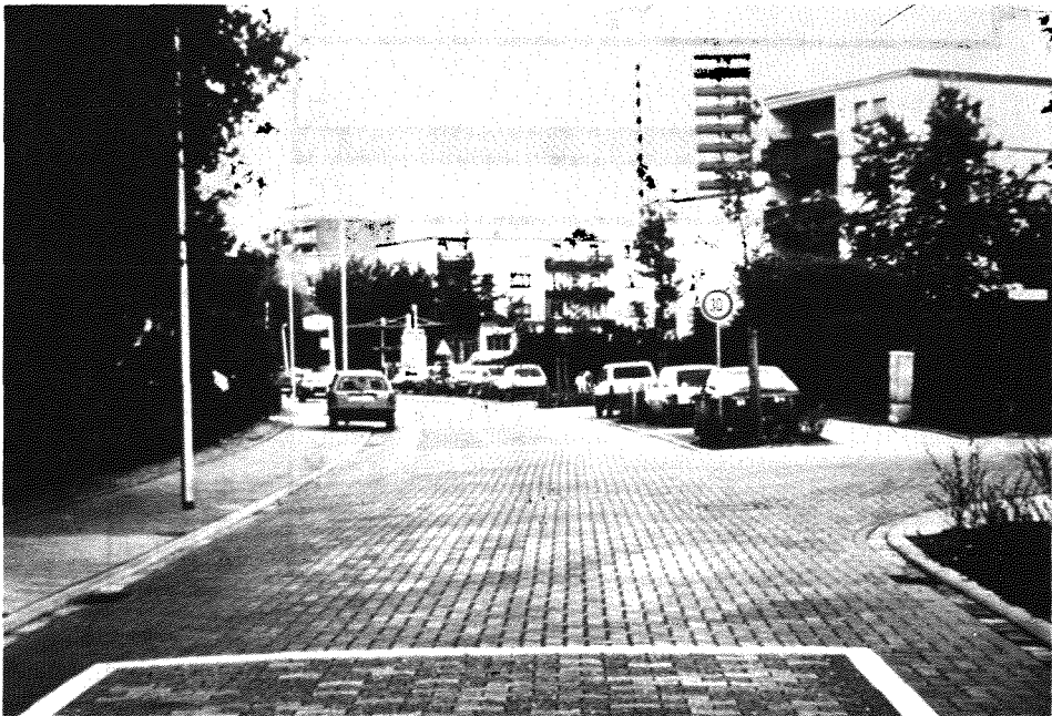
Figure 12b: A residential street after reconstruction (Buxtehude)
