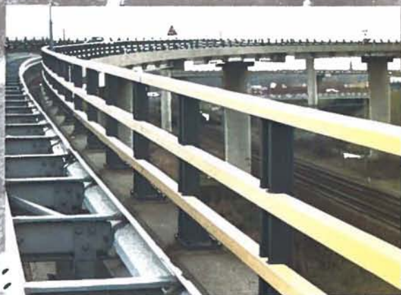
Safety barrier and safety fence
