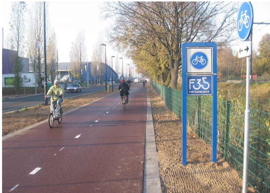
Figure 8. Example bicycle highway (Photograph: Fietsberaad).
