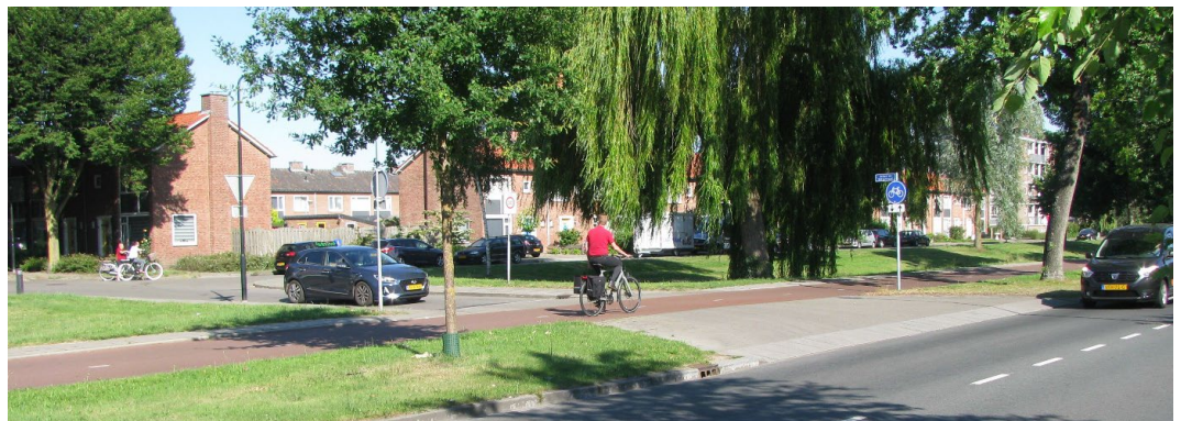
Figure 11. Two-way bicycle track with a cyclist coming from the right side from the perspective of the side road of the main road where a cyclist crosses a side street and may be overlooked by drivers coming from the side street (Photograph: Paul Schepers).
