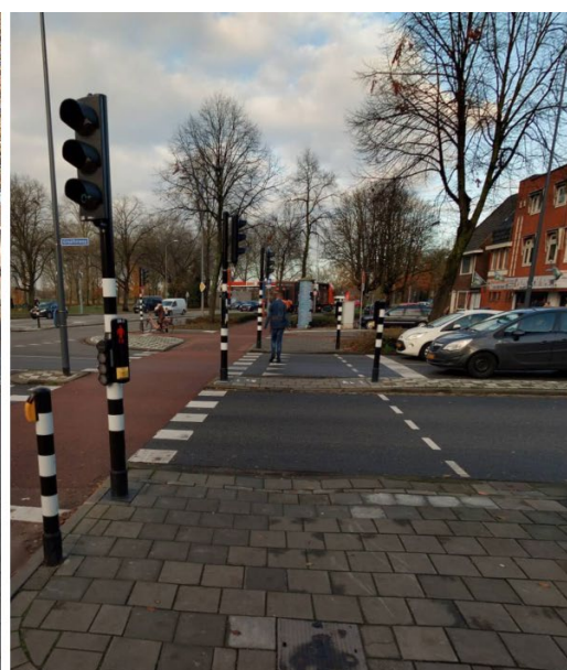
Figure 5. Above: pedestrian light at the beginning of the crossing, the 'Maastricht position' (Photograph: Eric Greweldinger). Below: Before and after installing pedestrian lights at the 'Maastricht position' in the city of Den Bosch (Photograph: Cyclomedia).
