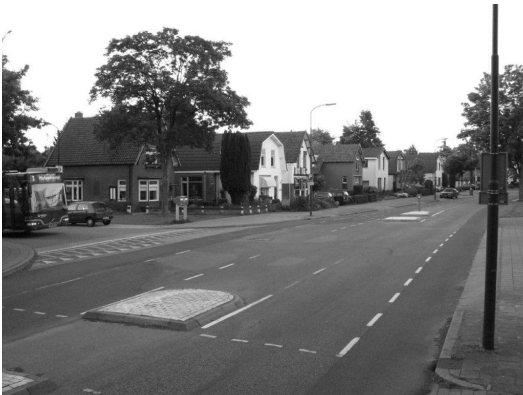
Figure 4.2. Example of a bicycle lane for through cyclists, an exit construction at minor roads and raised middle islands that enclose a left-turn section for both cars and cyclists crossing the two-lane priority road.
