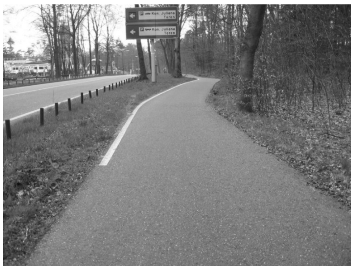
Figure 6.2a. Bicycle path delineated with a clear edge-of track marking.
