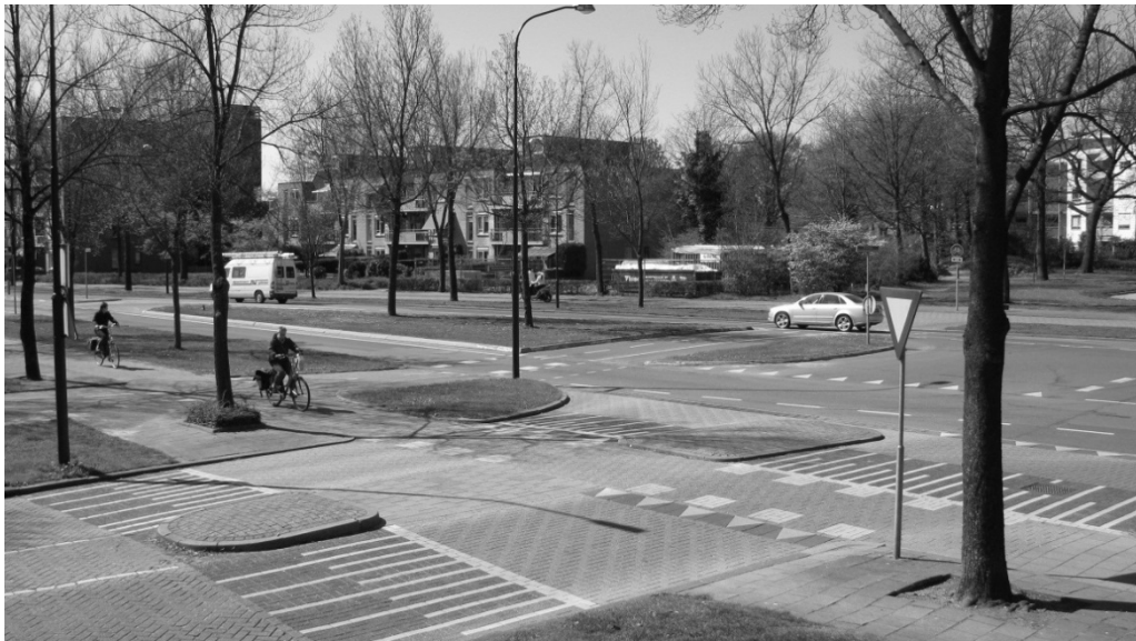
Figure 4.1. Example of a well-marked, raised bicycle crossing for through cyclists on a one-way cycle track with a distance of over five metres from the priority road; a raised middle island with a separate space for cyclists crossing the two-lane priority road.
